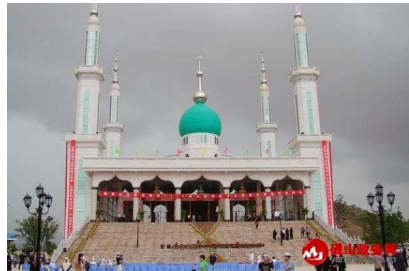
Songmaopo Mosque before the renovation project. Source: baike.com
